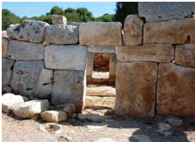
Figure 4. Quarried limestone blocks. (a) Equidimensional to tabular blocks in Cartailhac Building. (b) Elongated rectangular vertical uprights used possibly to support the roof of the structure; square ashlar stones are visible along the back walls.
