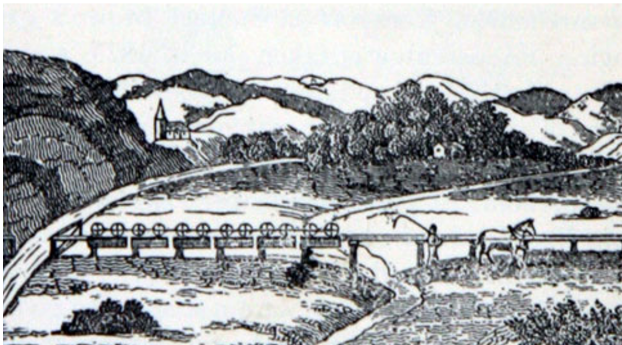
Figura 2. Monorraíl Palmer (1822) en un terreno irregular. Grace's Guide To British Industrial History. Henry Robinson Palmer.
