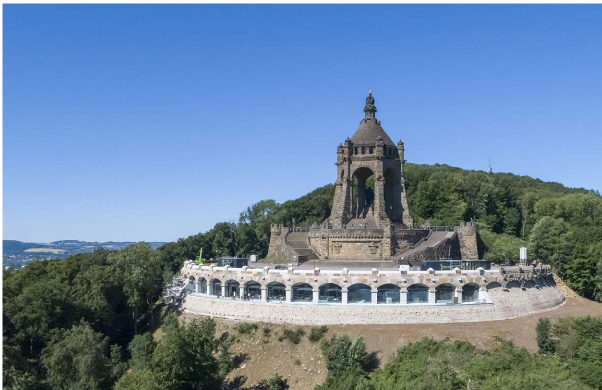
Figure 4. Monument Kaiser Wilhelm at Porta Westfalica with original brown Porta sandstone at the monument and new white Obernkirchen sandstone at the wall (photo Peter Hübbe).
