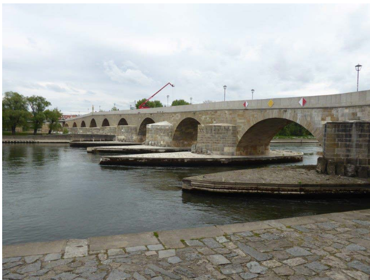
Figure 7. Stone bridge in Regensburg after restoration with new granite railing (photo Klaus Poschlod, 2018).
